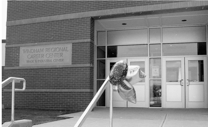
Front of Windham Regional Career Center building.
